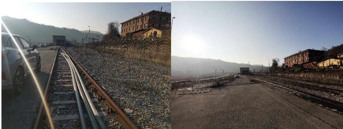
Figure 10. Rail tracks available at the site
