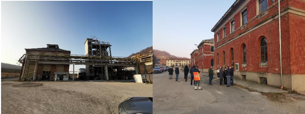
Figure 11. Residual plant – Two-level buildings
