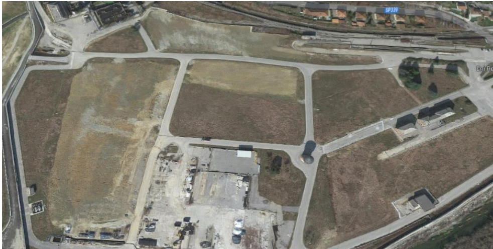
Figure 13. Internal road network
